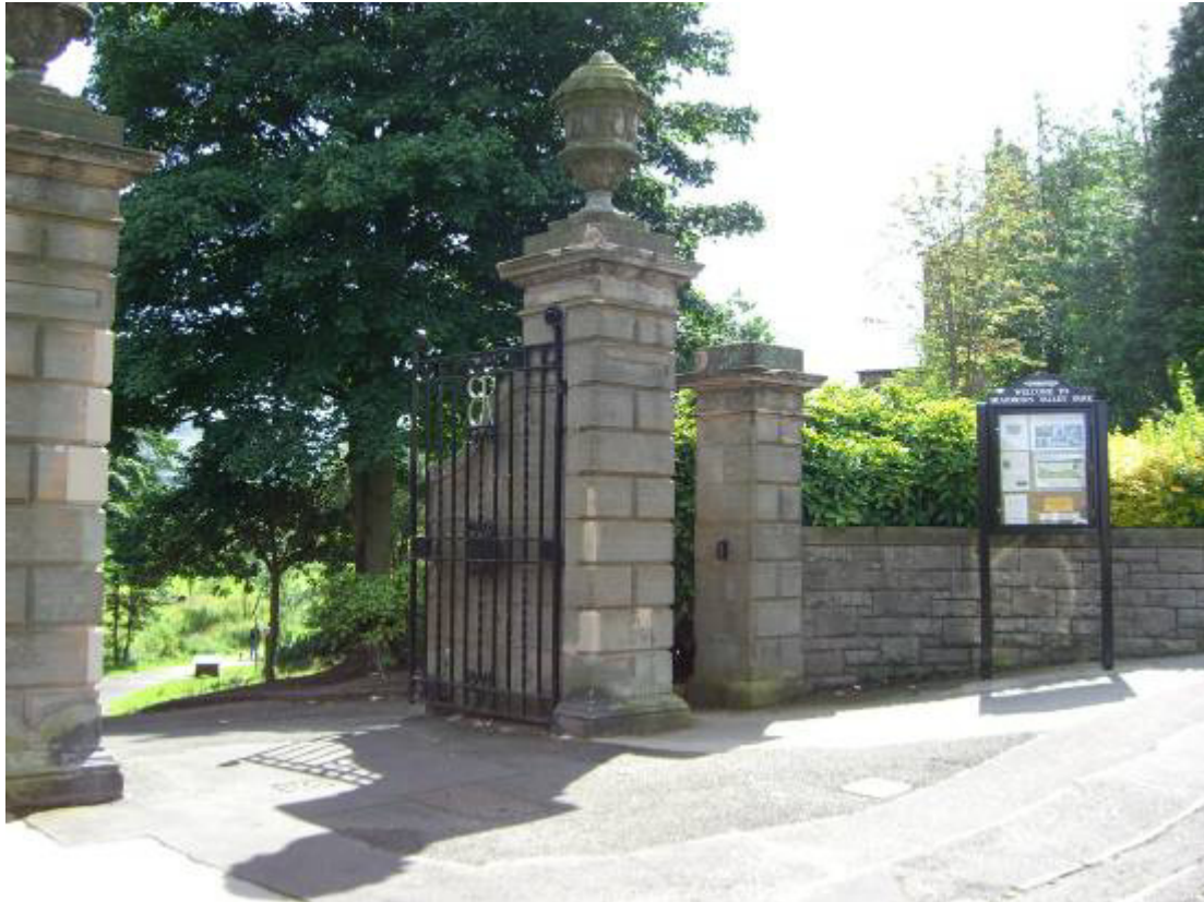
Main Entrance to the Park.
